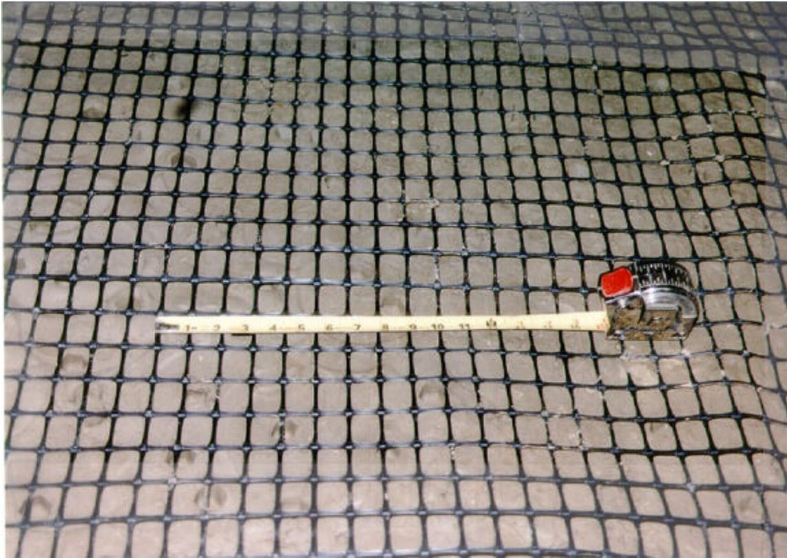
**Figure 2. Geogrid Reinforcing On Compacted Soil Lift.**
