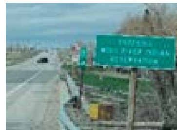
Current Portal Entry
