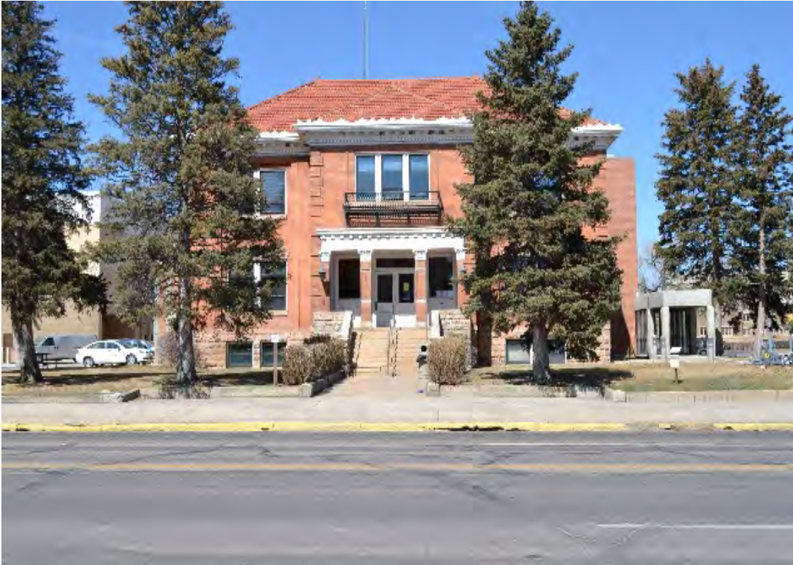
Photograph – Laramie Carnegie library building adapted for new use, 2013. Richard W. Waggener photo, Waggener family archives.
