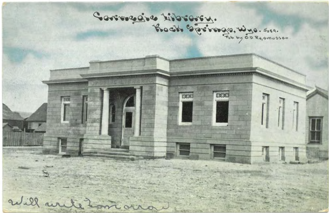
Photograph – Rock Springs Carnegie library, year unknown. James L. Ehernberger Western Railroad Collection, 1849-2016. Box 720. American Heritage Center, University of Wyoming.
