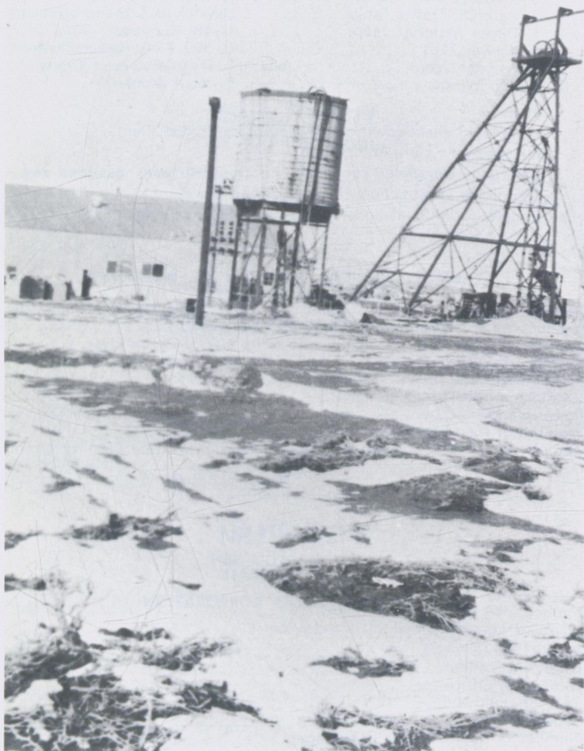
Head Frame and Construction at the new shaft, Allied Chemical Company located 19 miles West of Green River, Wyoming.
