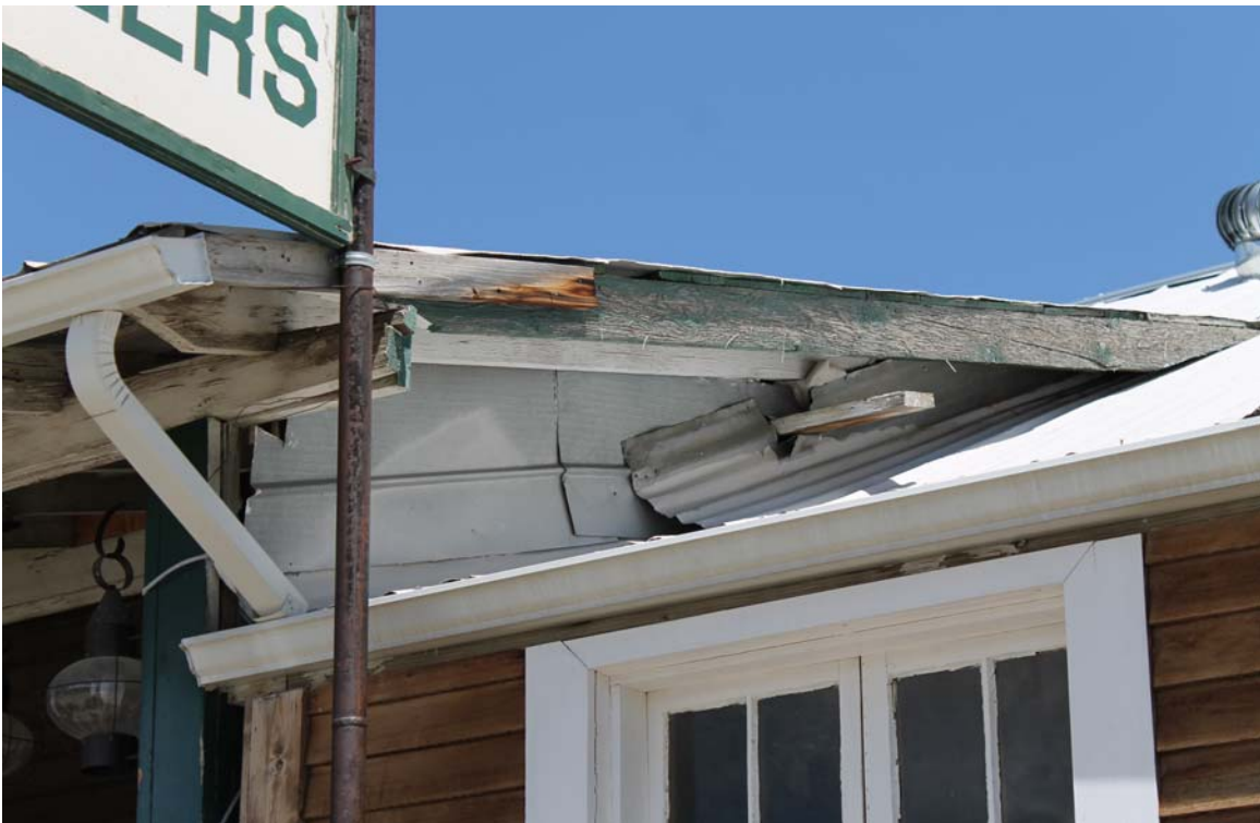
Photo 6: Roof pitch change at the Kitchen and Front Entry.
