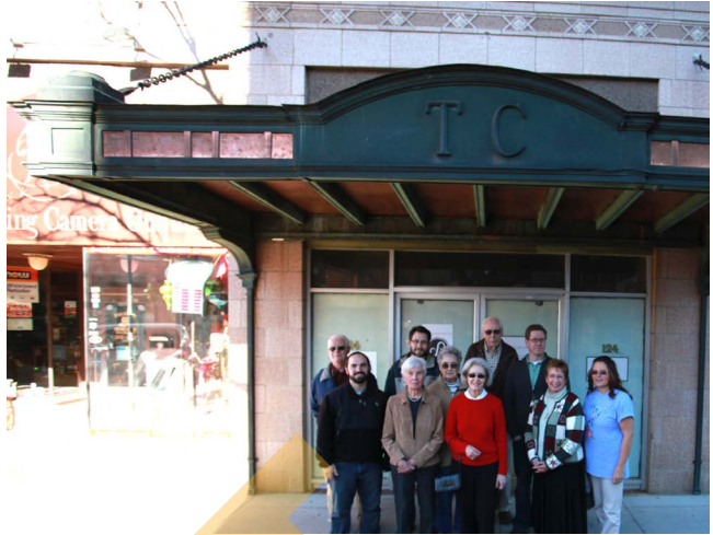
The Casper Historic Preservation Commission members meet at the Turner-Cottman Building to inspect the copper awning which was recently restored by the owner. If a National Register Historic District is established in Casper, the property owner will then be eligible for historic tax credits for this and future renovations to the building.
