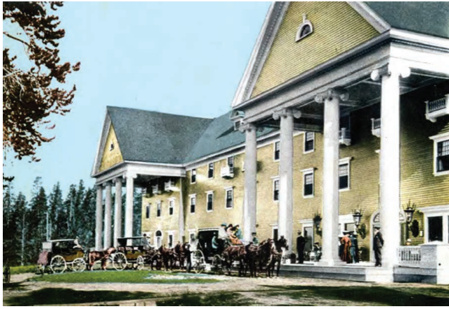
From draft NHL nomination form: In 1903, the Yellowstone Park Company hired architect Robert Reamer to prepare designs to enlarge the Lake Hotel. As part of Reamer’s design proposal, the hotel was transformed into a notable work of Colonial Revival architecture that featured large porticoes, columns, and a symmetrical principal facade. View, circa 1920. (Source: Yellowstone Photo Archives, National Park Service, YELL 30212)
