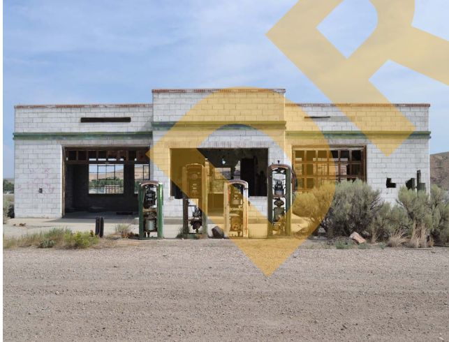
Abandoned Sinclair station on U.S. 30, Jamestown. Photograph by Beth King.
