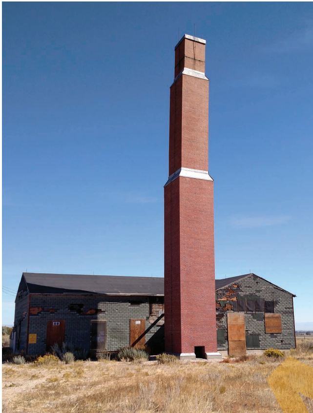
Heart Mountain Boiler House Chimney. Photograph by Mary Hopkins.
