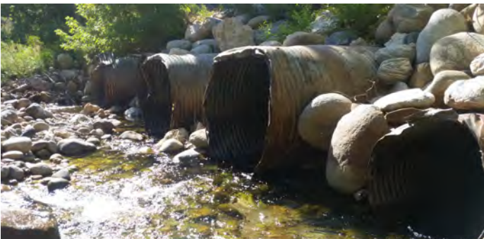
The problem: four 5-foot wide and two 3-foot wide culverts
