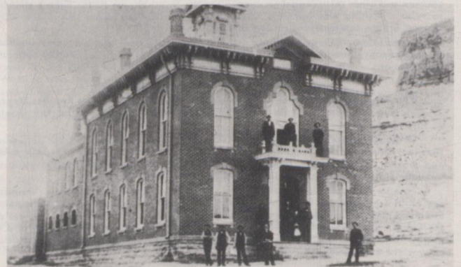
Sweetwater County Court House was built in 1876 at Green River
