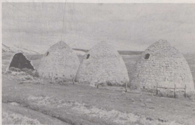
These 30-foot tall antique kilns once supplied the iron industry of Utah with the charcoal fuel needed in smelters
