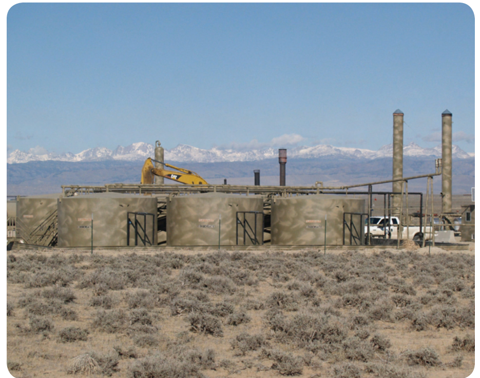
Camouflage paint technique used to reduce visual impacts to the setting of the Lander Trail, Sublette County.
