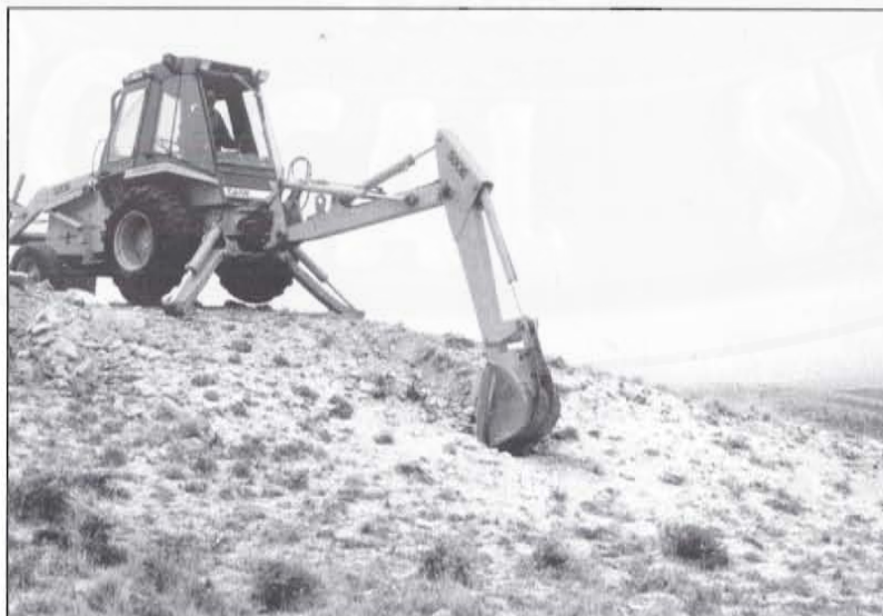
Figure 4. Volcanic ash outcrop (backhoe beginning to dig trench 1).
