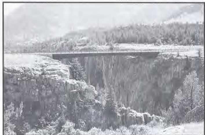
Figure 33. Bridge over Sunlight Creek viewed from the west. Cambrian rocks are exposed in the low tree-covered hills behind the parking area to the right; Precambrian rocks are exposed in the canyon and on either side of the bridge. (Photograph by WDOT, Geology Program, 1994.)
