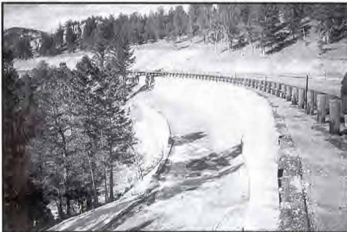
Figure 29. View to north (before third switchback) of Three Forks and Jefferson Formations. Klippe of Madison Limestone exposed above road level in upper left part of photograph. Note retaining walls of geogrid blocks. (Photograph by WDOT, Geology Program.)
