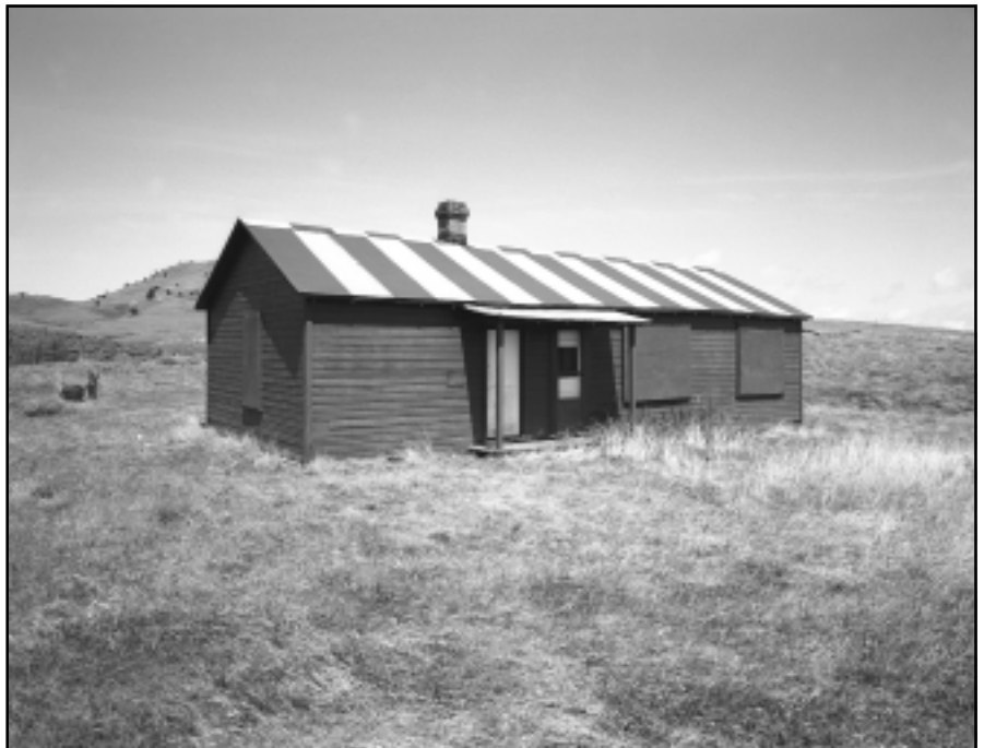
Bunk House, F.S. King Brothers Ranch Historic District, Near Laramie. Photo by Richard Collier.
