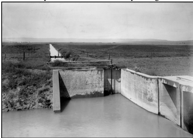
Shoshone Reclamation Project
