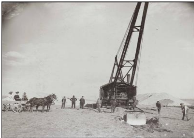
Lake Hattie Dam Construction
